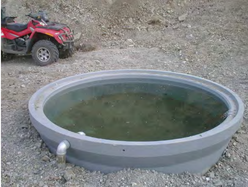
This large circular concrete trough will provide clean water to the livestock that have been fenced away from the creek. The large circular concrete troughs are the most common installed in Baker County. They are known for their longevity and durability.
