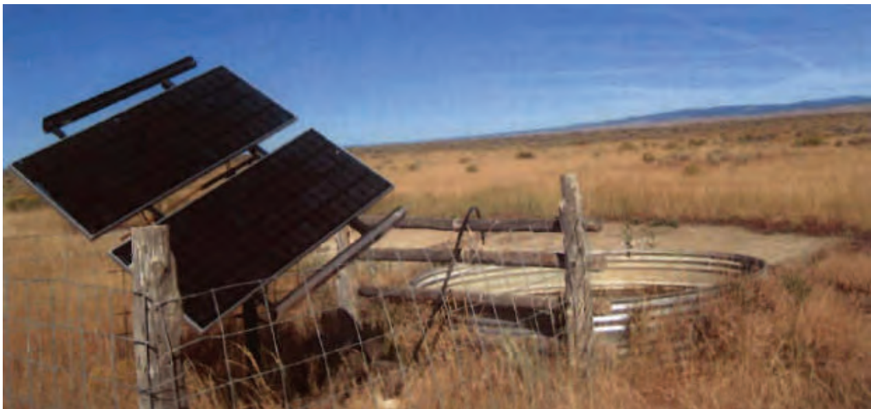
A solar panel provides power to pump water to a trough for livestock and wildlife drinking water on the Starbuck Ranch in Harney County. The new water source helps manage livestock grazing, allowing native plants to regenerate.
