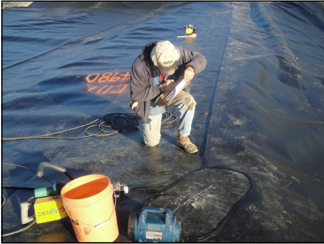
By installing the cover, Heard Farm owner, Dick Heard, could avoid adding more aerators to his lagoons and avoid greatly increasing his electricity use.
