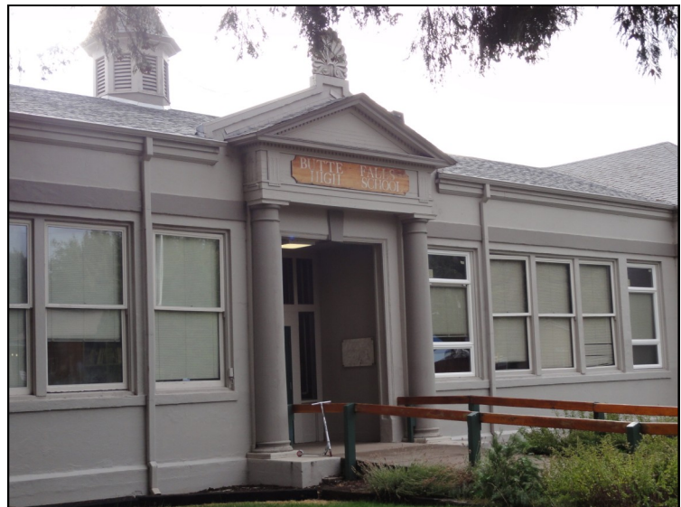
Butte Falls School District received $125,000 in Recovery Act (stimulus) funds for a new energy-efficient boiler and insulated pipes. The Oregon Department of Energy awarded the funds in a competitive solicitation.
