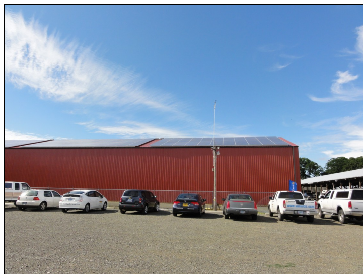
More than 300 solar modules sit on the roof of the new Benton County Fair Livestock Building. The modules were paid for with stimulus funds from an Energy Efficiency and Conservation Block Grant awarded by the Oregon Department of Energy. The new Fair Livestock Building was paid for with funds raised by the Benton County Fairgrounds Foundation. The new building houses a Solar Education Center.
